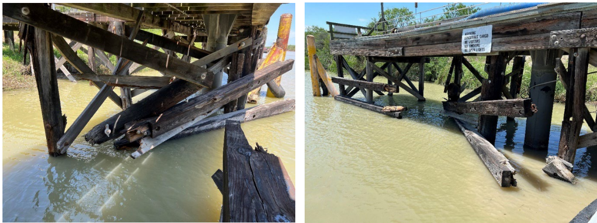
Figure 3. A 2023 barge strike damaged one of the Port's main docks making the infrastructure unsafe for barge operators and dock workers to utilize. Even with temporary repairs, the dock is still only able to provide half its intended capacity.
