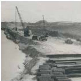
The turning basin is under construction (1951).
