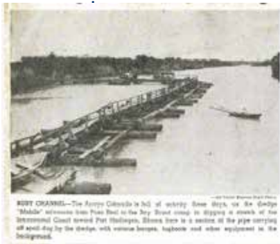
Dredging toward the Port site continues creating the navigation channel we know today.
