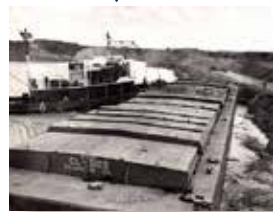
First barge of steel comes to the Port July 8, 1951. This was also the first barge to dock at the Port.
