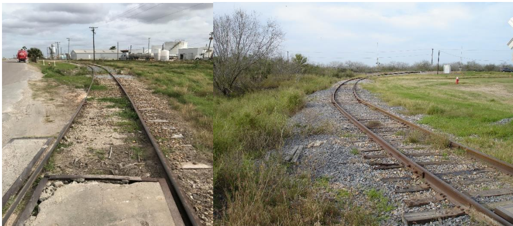
Figure 6 Existing Track Conditions
