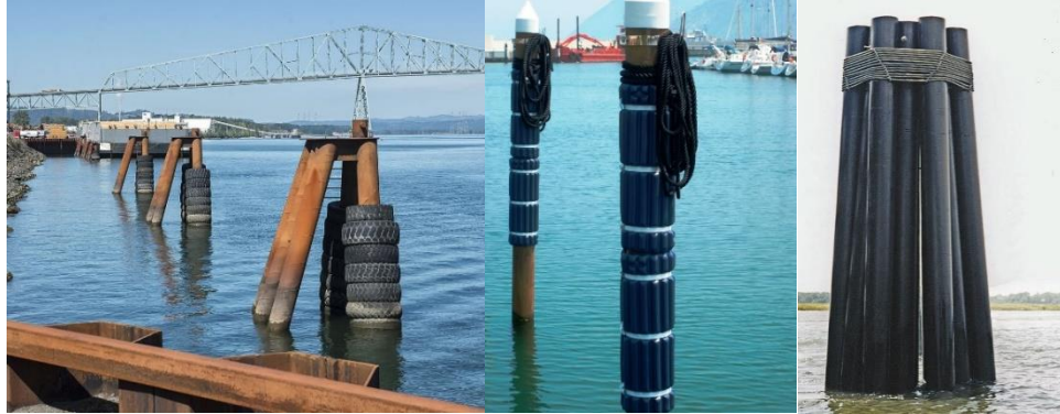
Figure 22 Mooring Dolphins-A Frame (Left), Steel and Synthetic Piles
