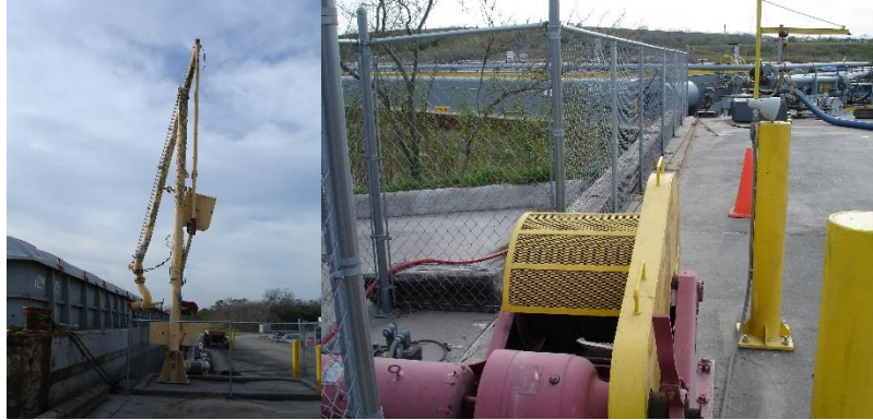
Figure 5 Liquid Fertilizer Loading Arm and Barge Mooring Winch
