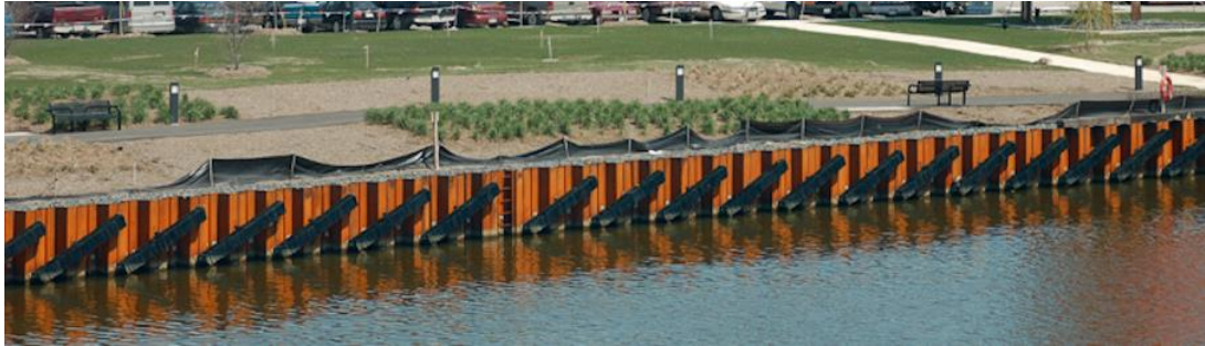
Figure 31 Sheet Pile Pier Construction
