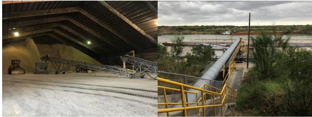
Figure 12 Sugar Warehouse and Conveyor System
